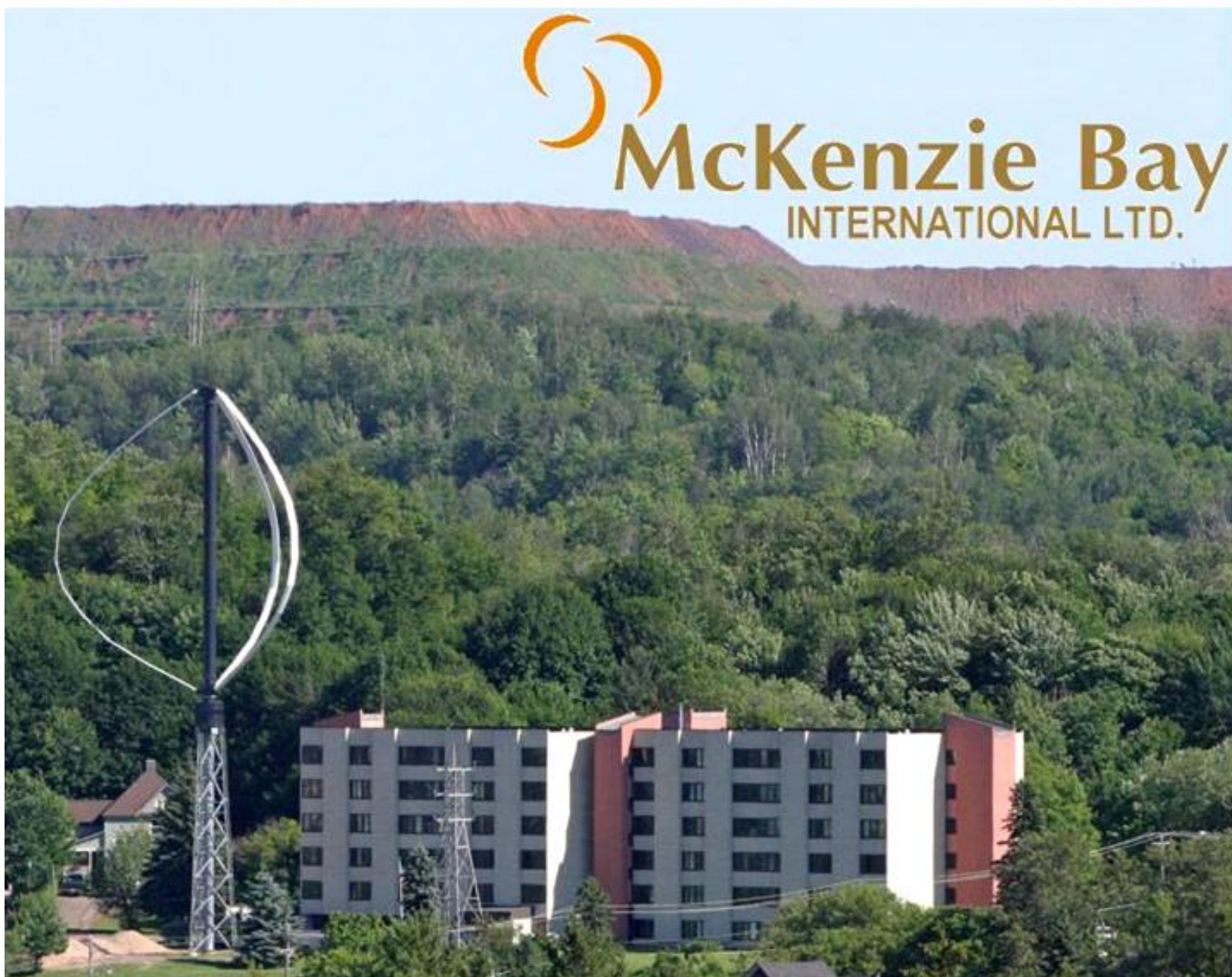
MCKENZIE BAY'S first WindStor vertical axis wind turbine was installed this summer in Ishpeming. Courtesy McKenzie Bay International
